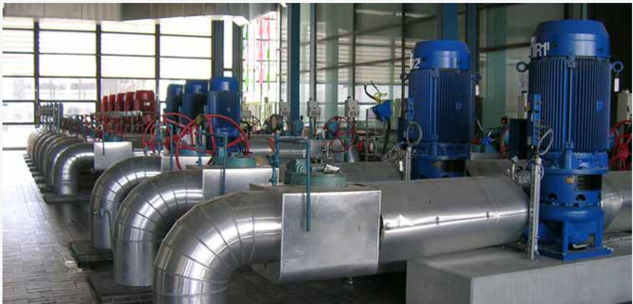
DESMI has supplied many pumps to this facility: Mainly vertical in-line centrifugal pumps model: NSL 200-415B/A12 & NSL 125-330 + 110 kW
